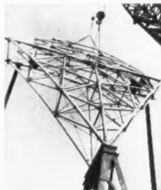
Steel beams support the first 50 x 75 ft pylon
